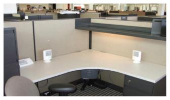
Figure 2. Johnson Controls Personal Environment Module with occupant sensor, control panel (on left), integrated task-light and desktop vents from underfloor air supply.
