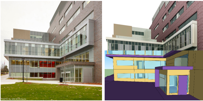
Figure 3. Real image (left), Revit model (top right) and BPS model (bottom right) of Canal Building
